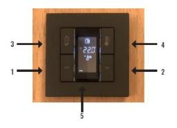
When the temperature in the room reaches that indicated on the thermostat, the radiator will turn off. It will start up again when the temperature falls below the temperature indicated on the display screen.
