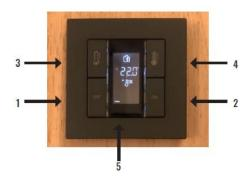
When the temperature in the room reaches that indicated on the thermostat, the radiator will turn off. It will start up again when the temperature falls below the temperature indicated on the display screen. Please contact our reception team if you have any doubts about its correct working.
